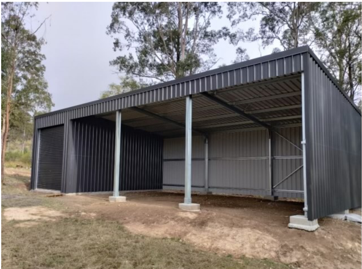
Figure 3 - View of Machinery Shed, constructed in 2024 as exempt development
