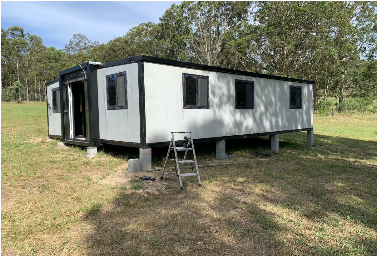
Figure 4 - Existing relocatable home to be used as temporary dwelling while principal dwelling is being constructed
